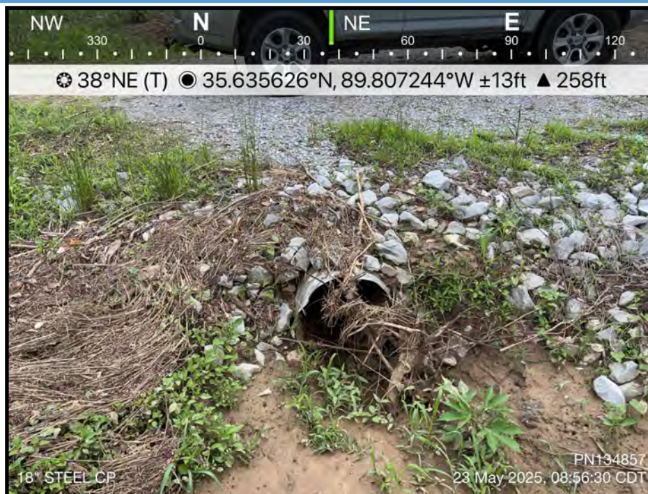
Photo 10: 18" Steel Corrugated Pipe—Farm field access across SR-87 from WTL-1
