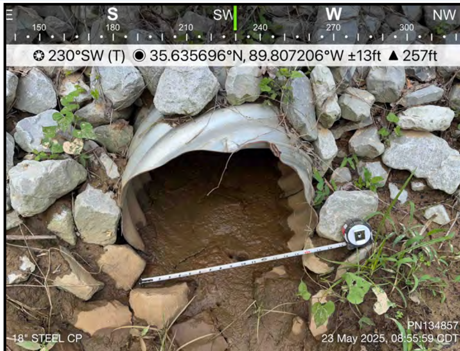
Photo 9: 18" Steel Corrugated Pipe—Farm field access across SR-87 from WTL-1
