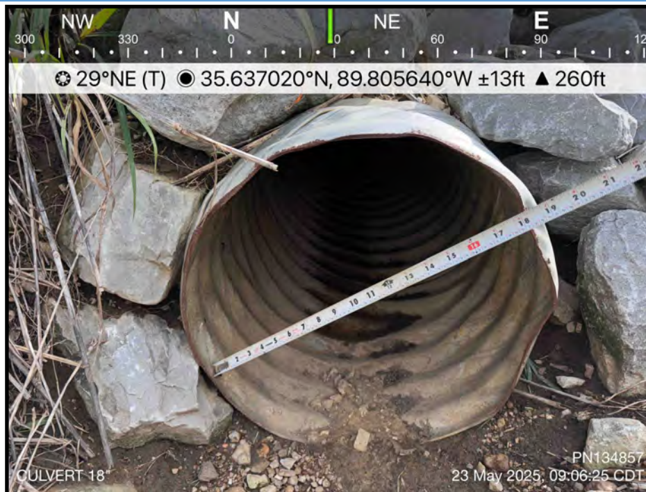
Photo 22: 18" Steel Corrugated Pipe—Farm field access over WWC-1/UDF-1
