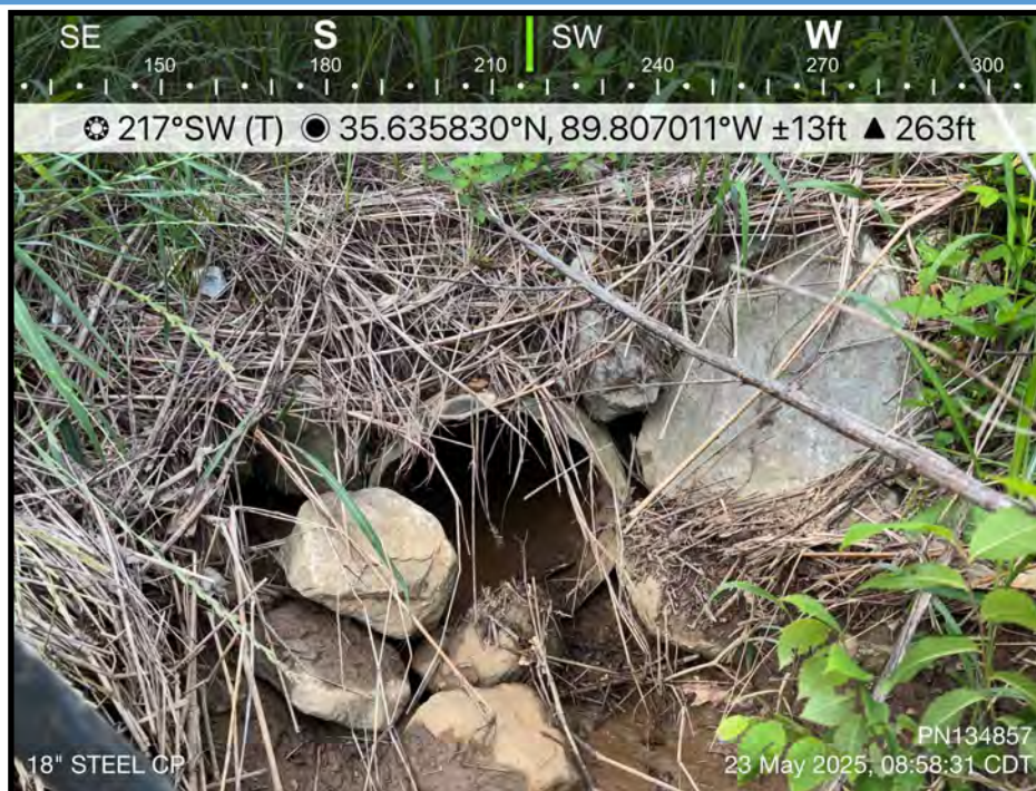
Photo 12: 18" Steel Corrugated Pipe—Farm field access across SR-87 from WTL-1
